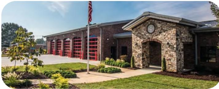
trusses, and for the bays a pre-engineered metal building. The roofing material is standing seam metal roof that will withstand the elements for many seasons.
